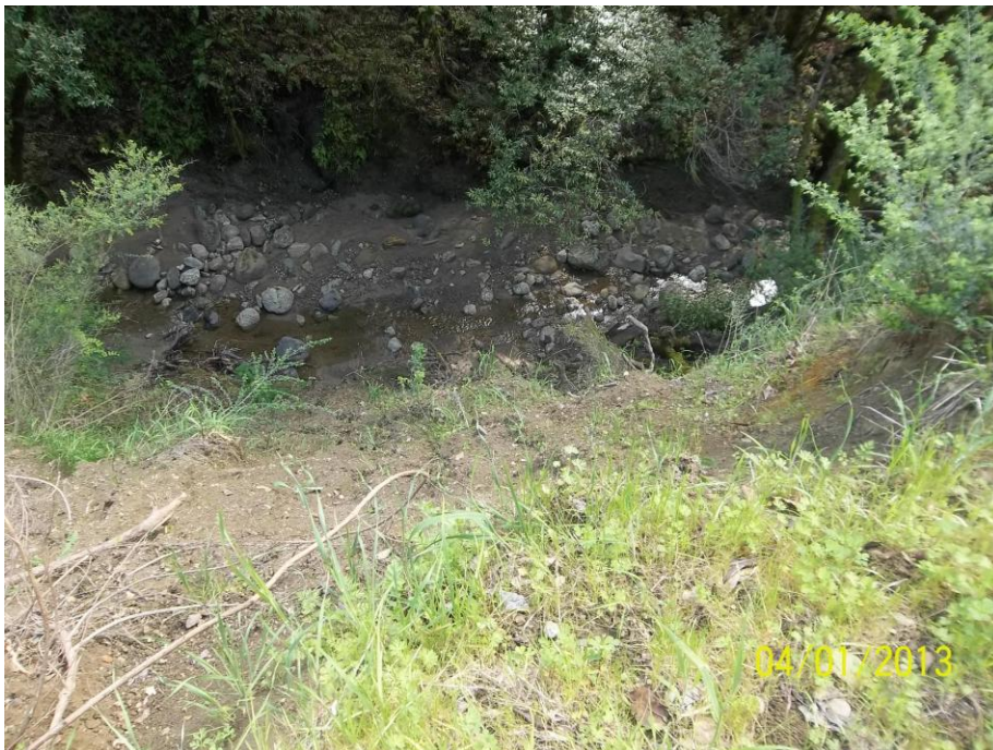
Photo 6 – Site 2: Photo showing near vertical drop from the roadway at the Site 2 slip-out located closest to the Joaquin Road intersection.
