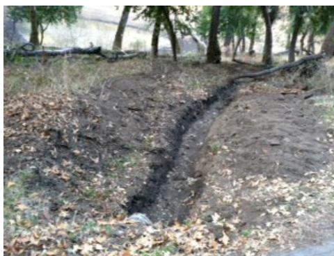
Trench leading rainwater outflow to Frog Pond
