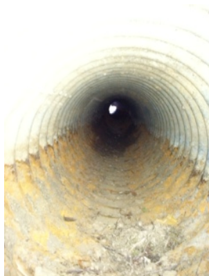
County cleaned-out pipe
